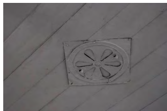
Figure 3.35 Ceiling detail showing ventilator.
