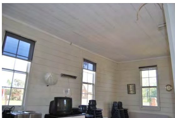
Figure 3.34 General view of the interiors of the Church Hall showing weatherboard walling, timber ceiling and double hung four-paned windows.
