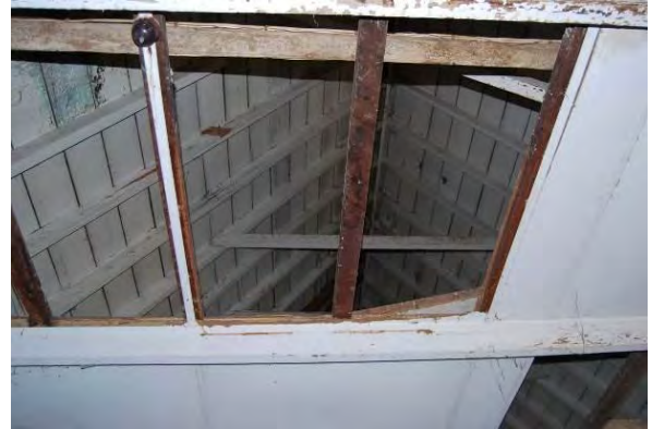
Figure 3.71 Interior view showing ceiling/roof detail. Note battens for shingles, and masonite ceiling covering. The roof is now clad in corrugated iron sheeting.
