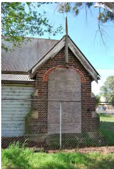
Figure 3.72 Detail of the gabled entrance porch on the south elevation. Note sandstone base and stepped ends, arched entrance and timber bargeboards and finial to the gable end.
