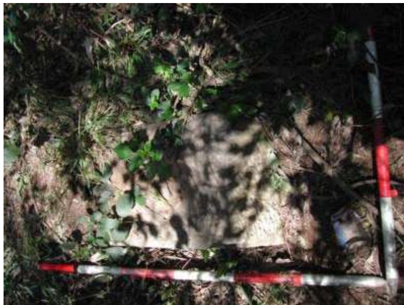
The east side of the culvert showing the collapsed top three courses. Despite the failure of the culvert, the sandstone blocks are still in good condition and should be reinstated.
