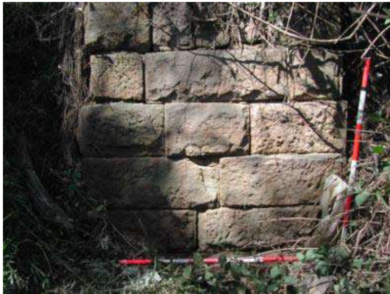
The west side of the culvert on Old Windsor Road south of Meurants Lane. Note the clay pipe in the lowest course beneath the range pole.
